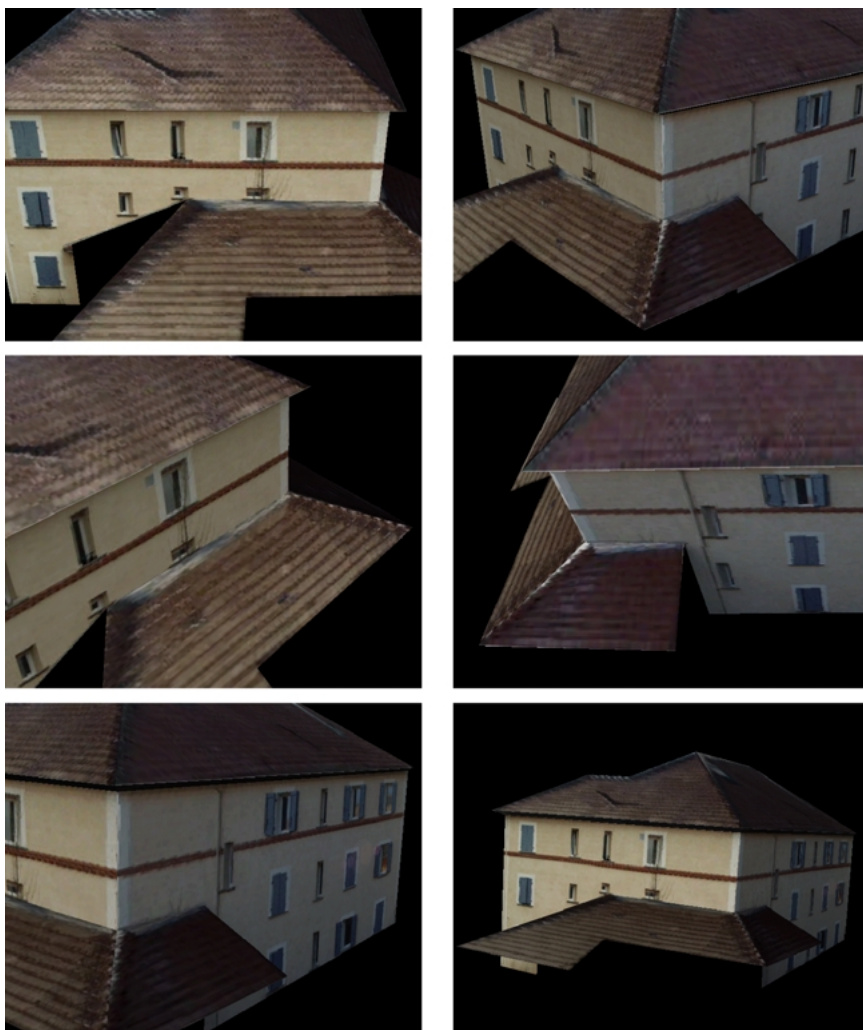
Figure 6. Different views of the textured model. Note that artefacts may be induced by possibly unmodeled non-planar parts of the surfaces, e.g. the pole bulging out of the roof in the top-right image is wrongly mapped to the roof plane, and is therefore distorted in other views, e.g. the top-left one.
