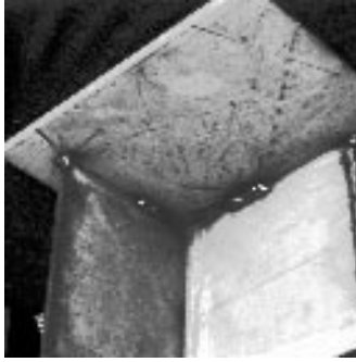
Figure 6: Detail of a part to be welded.
